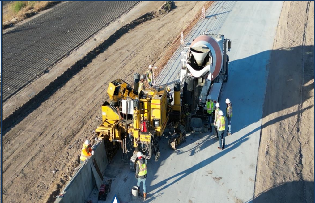
Single Slope Concrete Barrier
