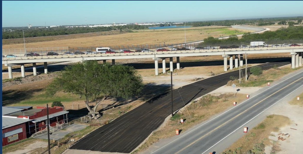
1" Bond Breaker/ Friction Coarse
